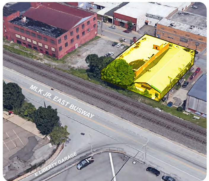
Site for potential new development
