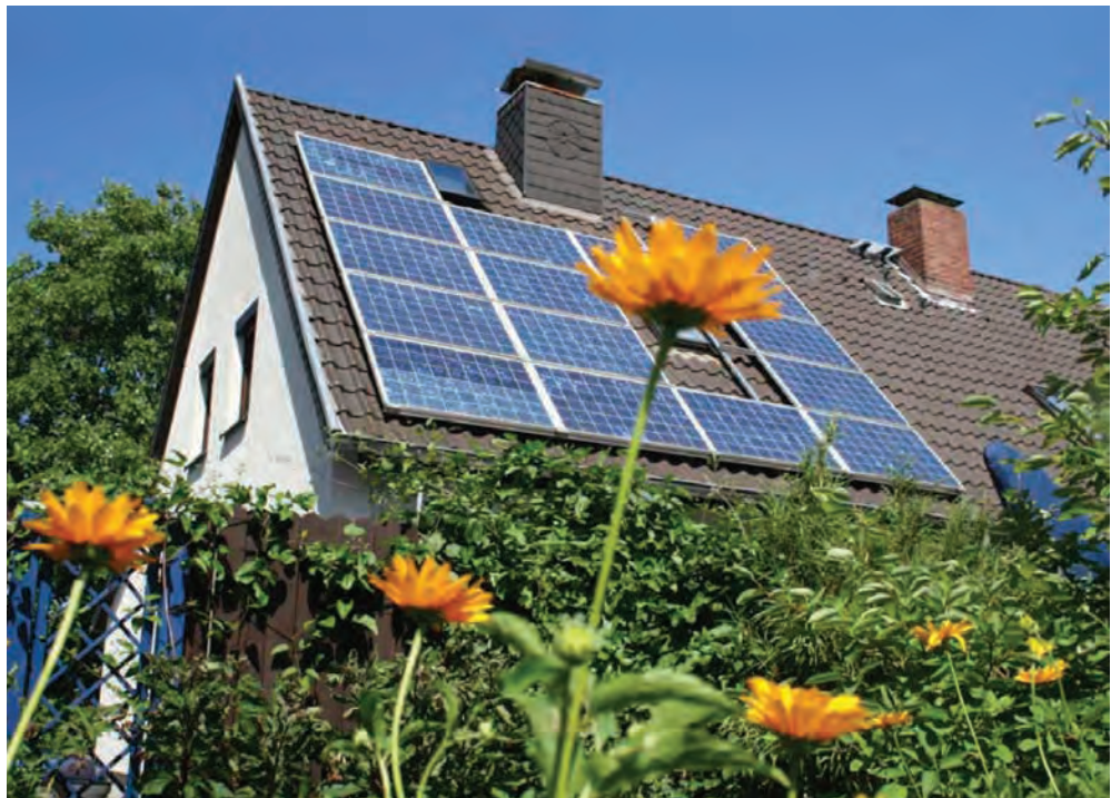
Fig. 28 Residence with solar panels
