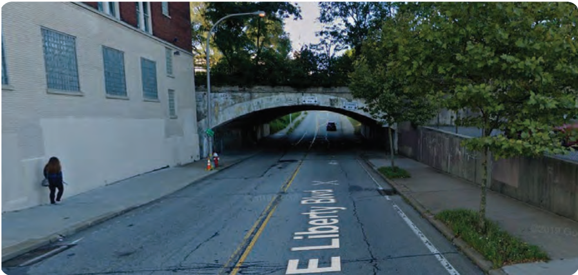
Site for improvement: East Busway underpass at East Liberty Boulevard
